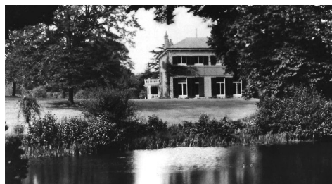
Keston Lodge, Croydon Road, in 1963 when it was a hotel just before demolition
